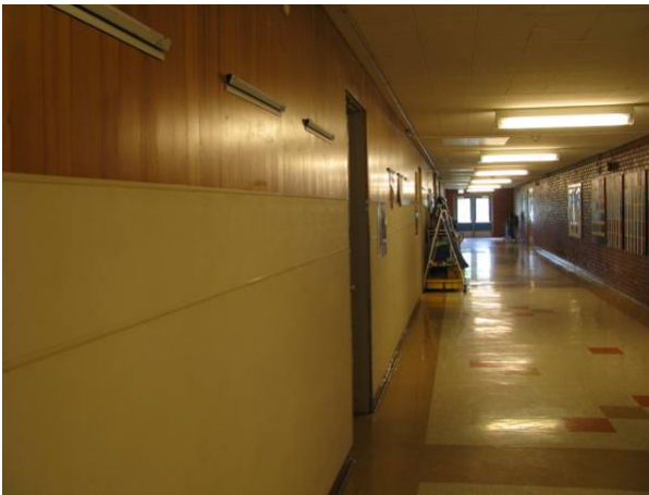
Building 234A corridor facing west
