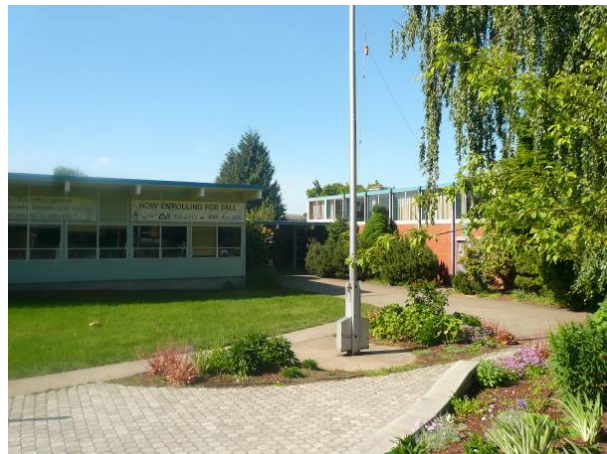
Entry to building 234C and 234A facing southwest
