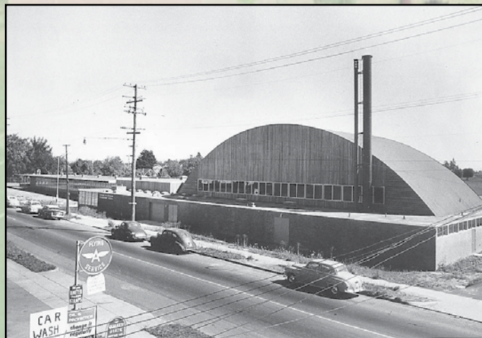
1950s photo showing gymnasium roof
