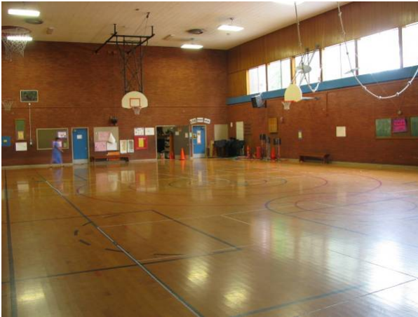
Building 234A gymnasium facing west
