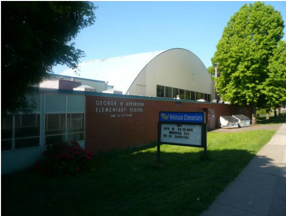
Building 234A facing southwest
